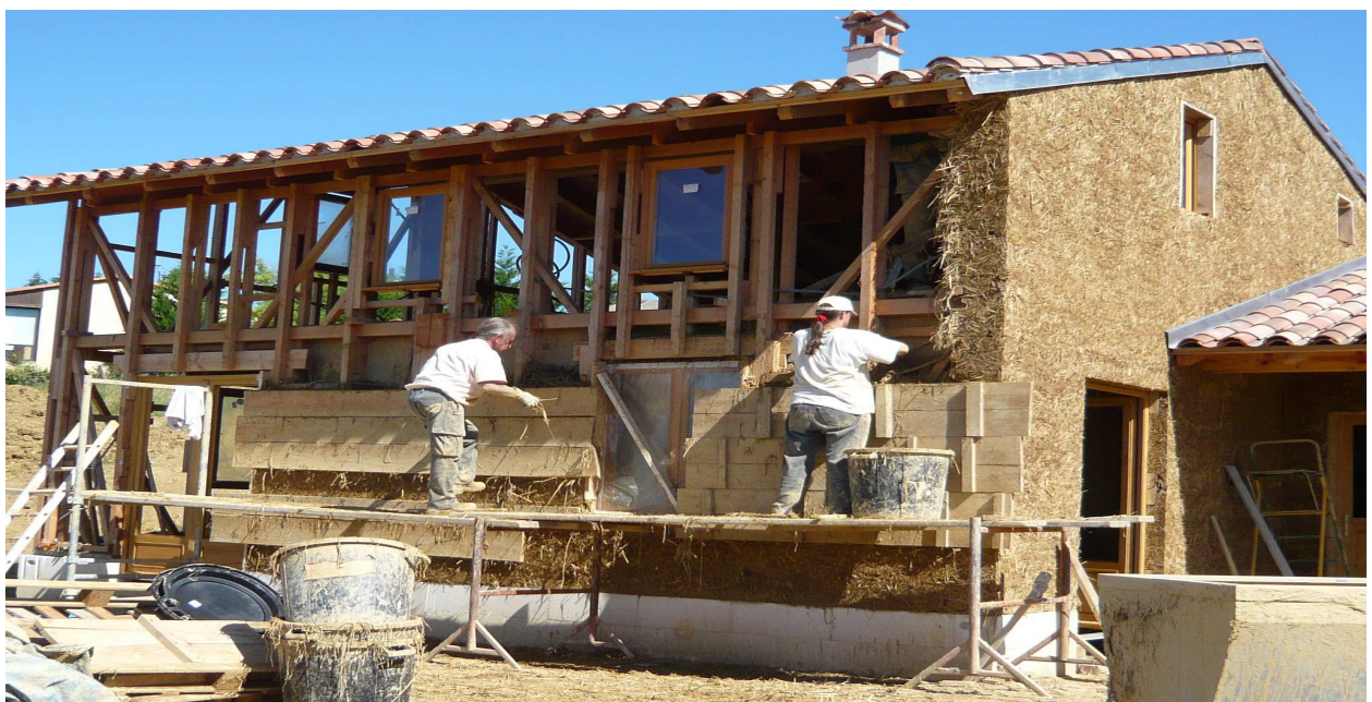
Figure 2: Southeast view: filling the walls with earth and straw
