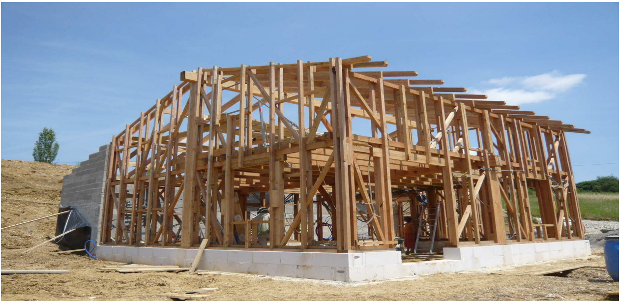
Figure 1: Northeast view: concrete blocks and cement concrete wall
